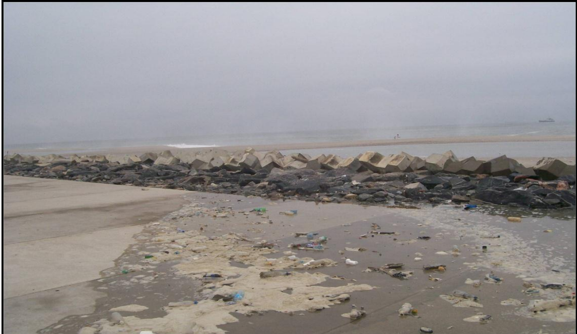
Plate7.3b: Storm surge control on Victoria Island, Lagos
